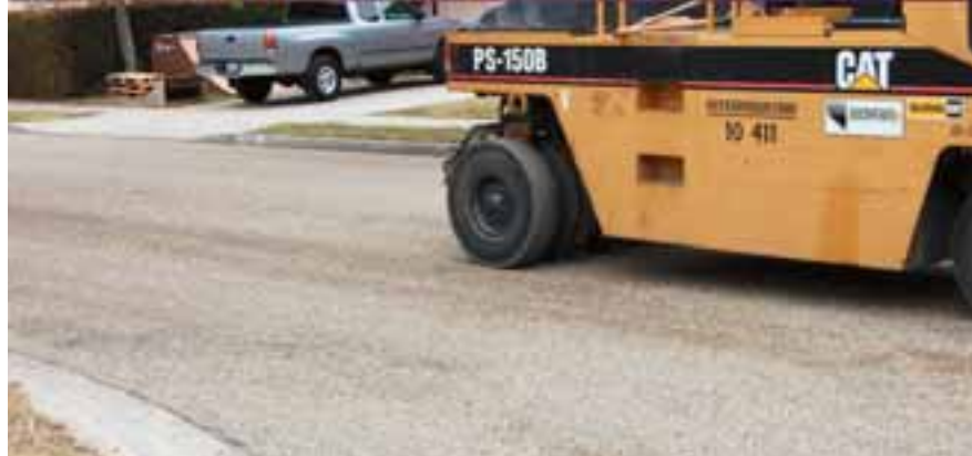
Aggregate is seated into PASS QB polymer modified emulsion on Santa Barbara County, Calif. local street, as part of county's award-winning program. Photo credit: Kevin Donnelly
