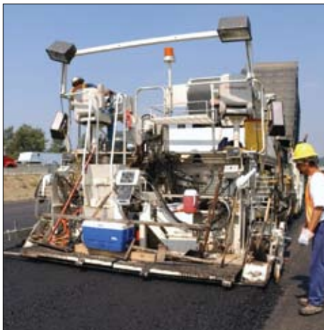
▲ Full-depth asphalt sections like hot mix asphalt perpetual pavements give portland cement concrete competition in long-term performance with minimal associated costs
