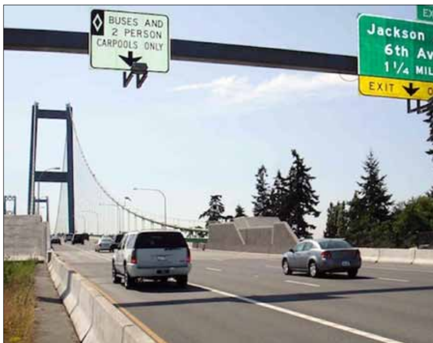
◀ Noise-suppressive barriers at cable anchorages on new Tacoma Narrows Bridge attenuate vibrating 'zipper' sounds from expansion joints.
