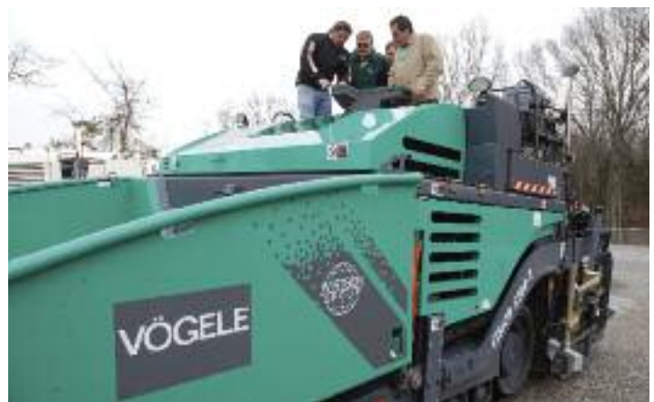
Then, same trainees see how system is used in real conditions in the field at adjacent Outdoor Demonstration Area
