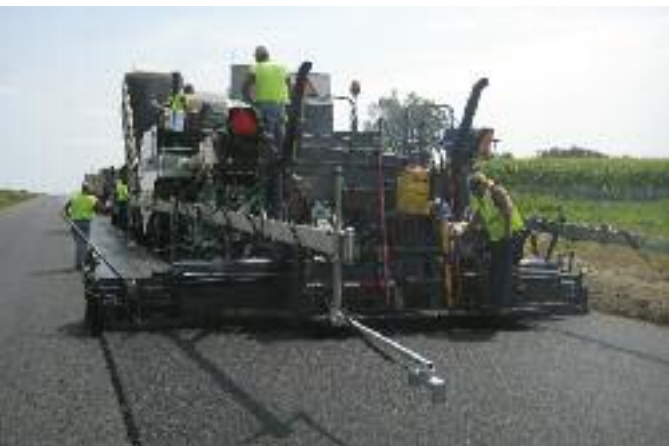
On Ohio 161, Shelly & Sands used dual 50-ft. sonic averaging skis to help eliminate longitudinal swales
