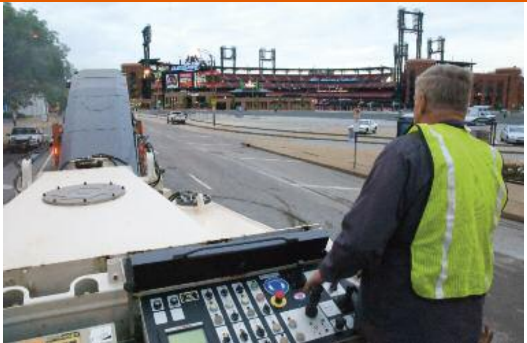
Operator Kenny Wencker mills just north of Busch Stadium using one of two W 2100s owned by City of St. Louis
