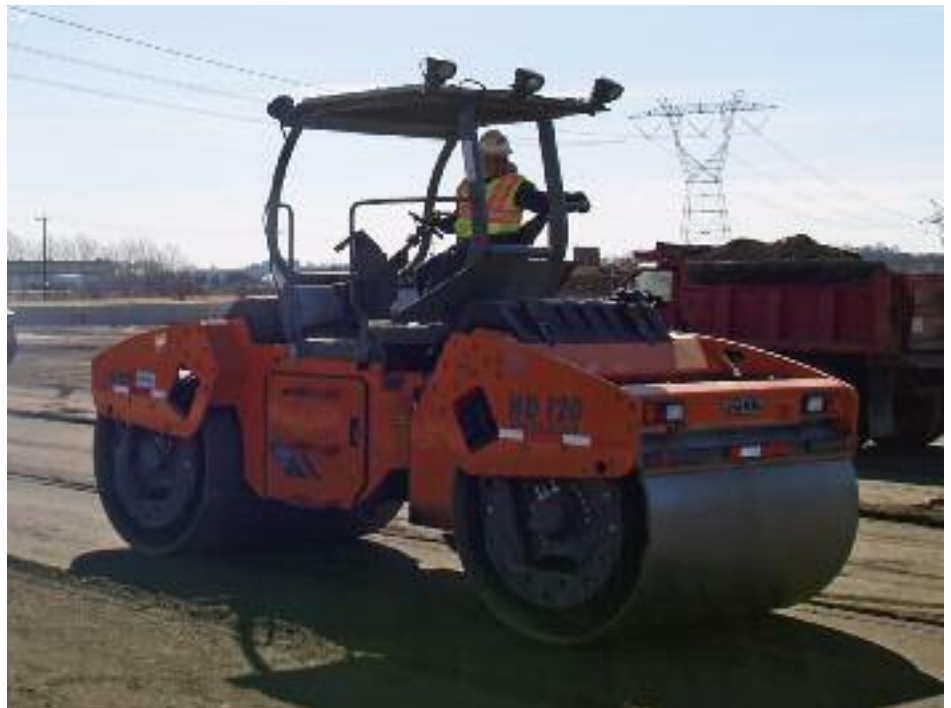
Local 825 operator gets experience in exclusive Oscillation compaction at union training facility using Hamm HD O120V
