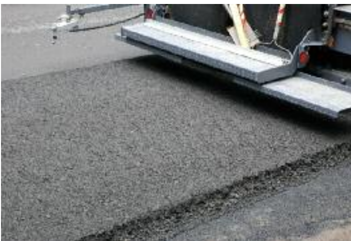
In Ulster County, N.Y., Reclamation Inc. was foamed asphalt-recycling the pavement surface "cold in-place" to a depth of 4 in
