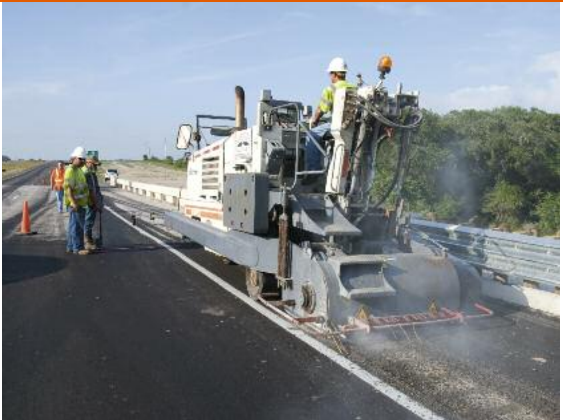
Larry Polasek operates W 600 with Rumbler III on U.S. 77; contractor PennTex achieved 40 percent increase in productivity with new Rhino bit design
