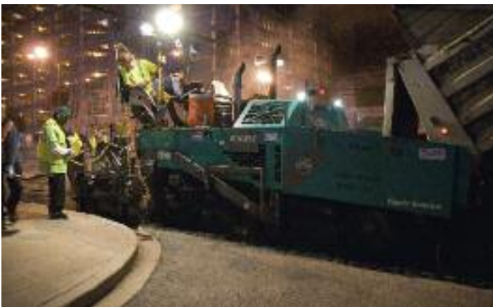
10-ft. Vögele America 2219T – predecessor to the Vision 5200-2 – places overlay across street from Busch Stadium
