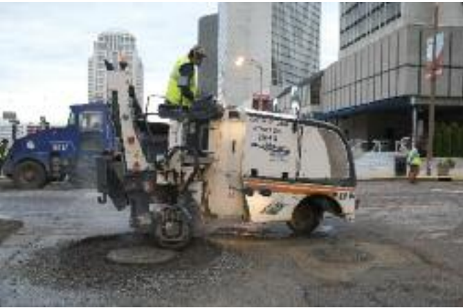
St. Louis' W 50 DC cuts around manholes but also does curb reveal
