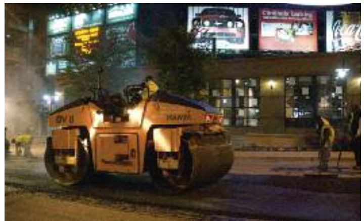
One of two of city's Hamm DV 8 compactors features split drums which city appreciates for rolling curves and intersections
