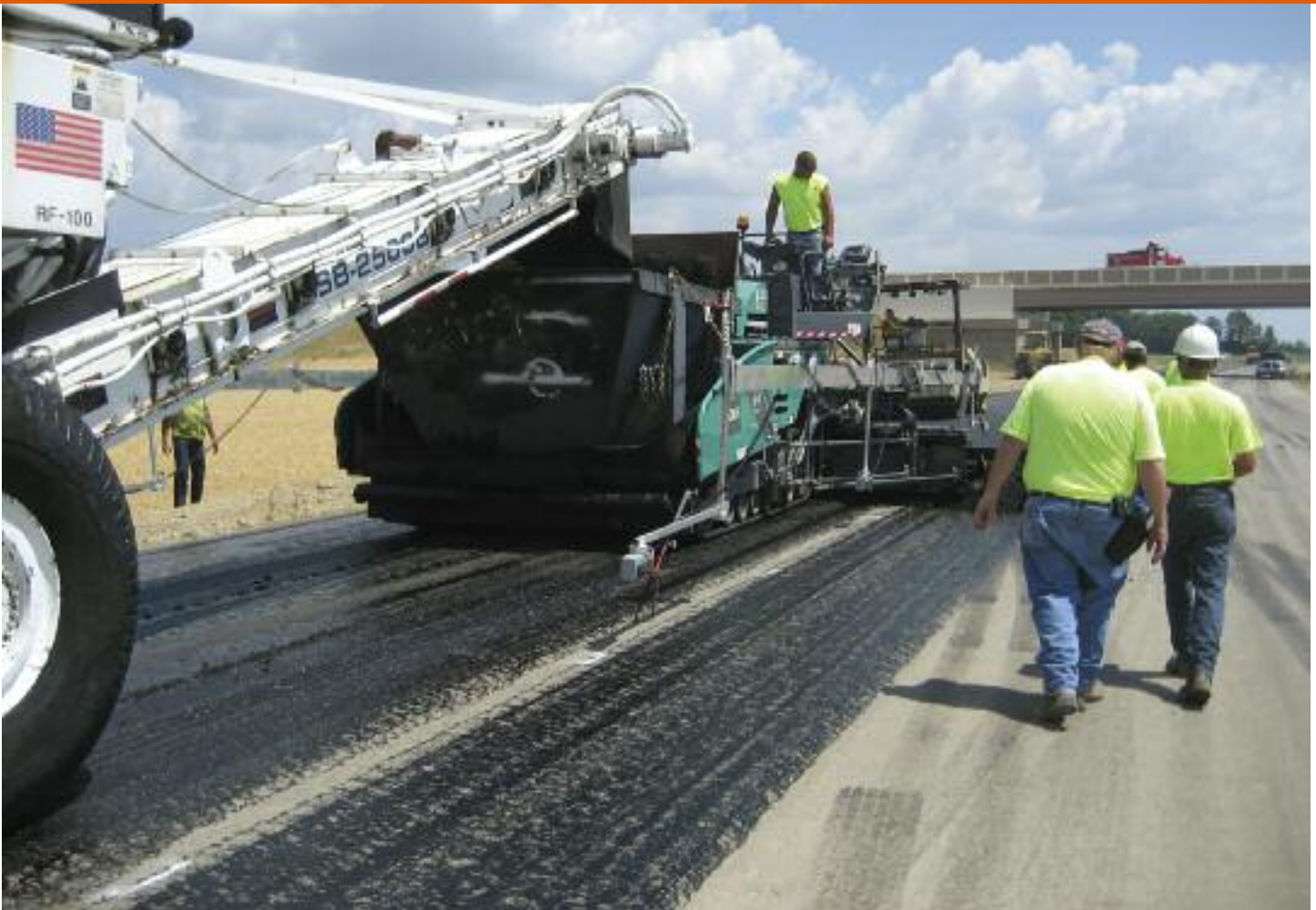
Shelly & Sands used material transfer vehicle at its option to control mix segregation and isolate paver from haul trucks, leading to smoother pavement
